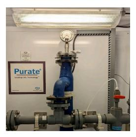
• Chlorine dioxide pressure transmitter went bad. This resulted in low vacuum alarms that prevent the generator from operating. A new transmitter was installed by Azure water solutions.
